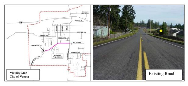
**Define the Problem:** Bolton Hill Road is built to rural standards with roadside ditches. It is lacking facilities for bike and pedestrian activity in an area with residential subdivisions and a sports complex/ball fields abutting the south side of the road. The residential side streets in the project limits already have curb and sidewalks and additional development is possible on adjacent vacant land.
